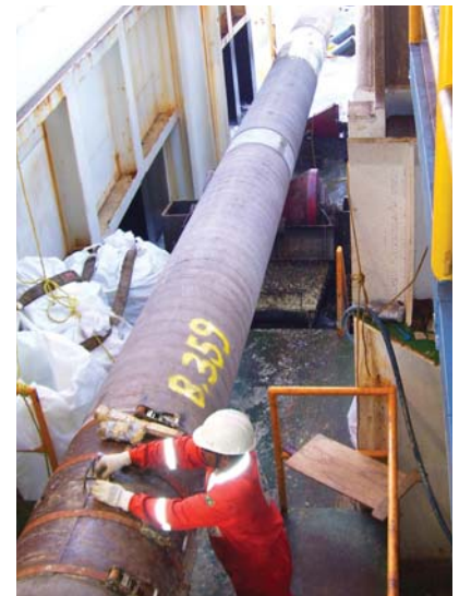
IFS field joints on gas pipeline
