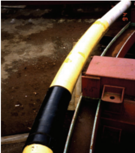
Solid Field Joint Testing
