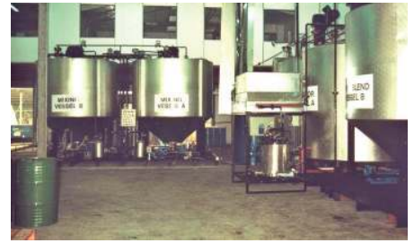
Malaysian NOP Plant
