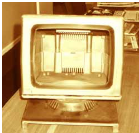
Figure 9 Television-back produced from Envirofoam 655
