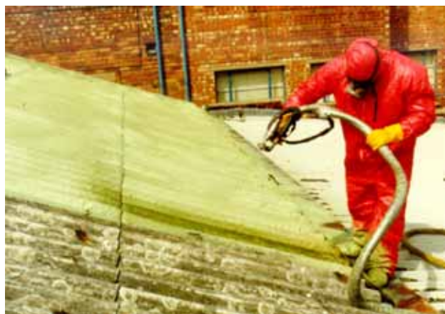
Figure 6 Spray-applied insulation based upon Enviropol 433
