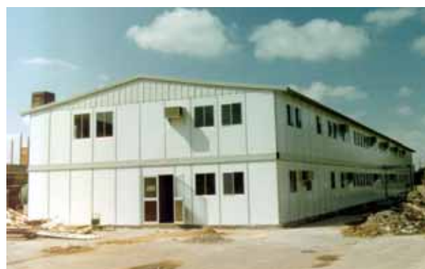
Figure 4 Insulated panels produced from rape seed oil based polyurethane
