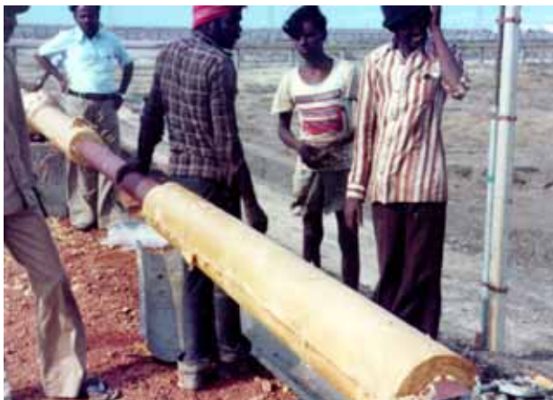
Figure 5 Pipeline being insulated with corn-oil based polyurethane foam
